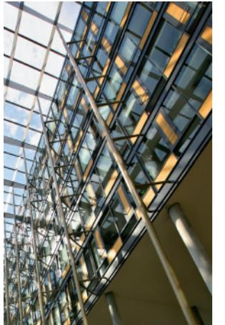
The atrium roof, made of ingeniously designed, grid-arranged beams of variable height, is supported by extremely slim pillars that are conically ended in contact with the roof; they amplify the subtle appearance of the structure. Stabilisation elements comprise heavy duty steel lift gears girders and cascade staircases and walkways hanging on pre-stressed ties. The glazed façades contain glass fins.
